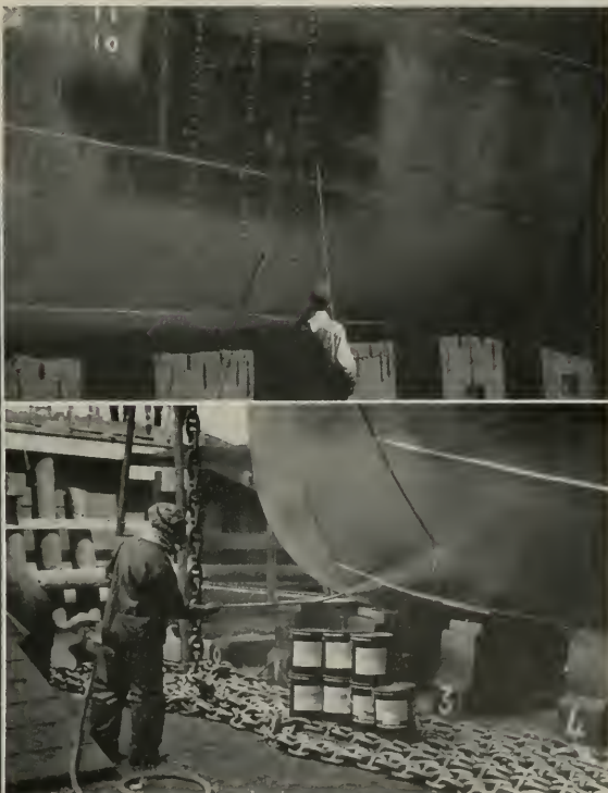
At right: Shipping Copper being applied to Pacific-Atlantic's Jose Pedro Verella. ▶
